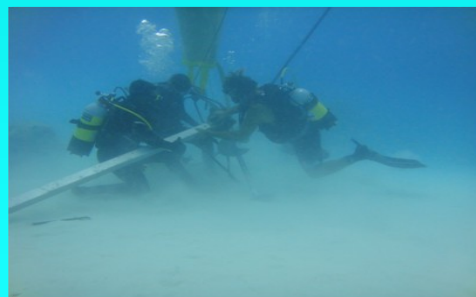
SNPA divers doing underwater drilling in sandy location
